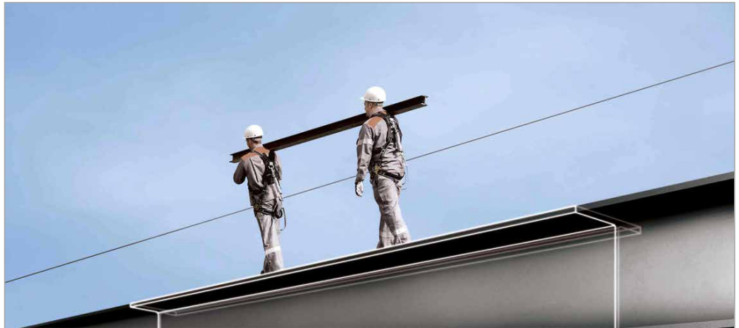
Employees on steel girders.
